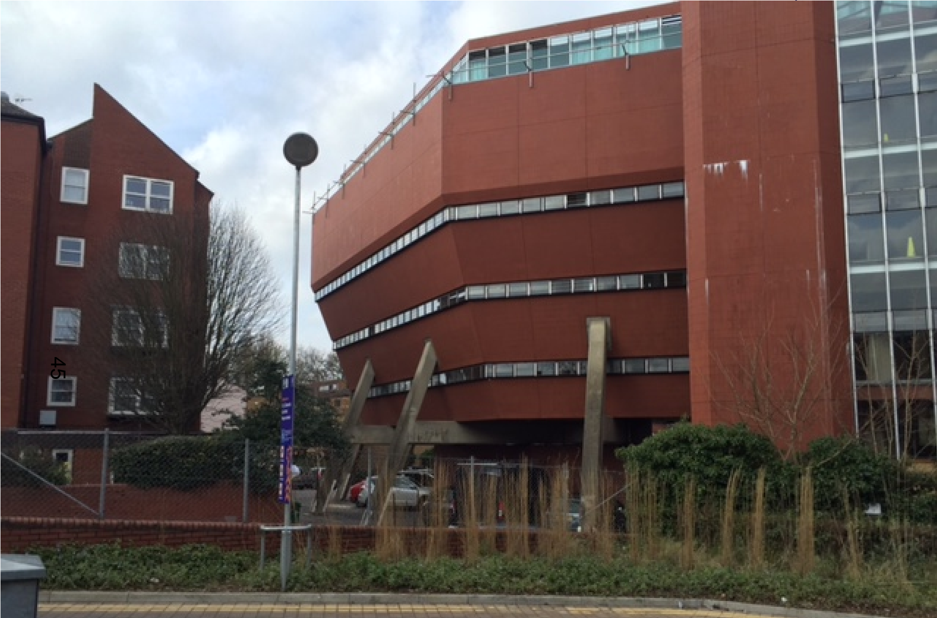
View of The Florey looking westwards
